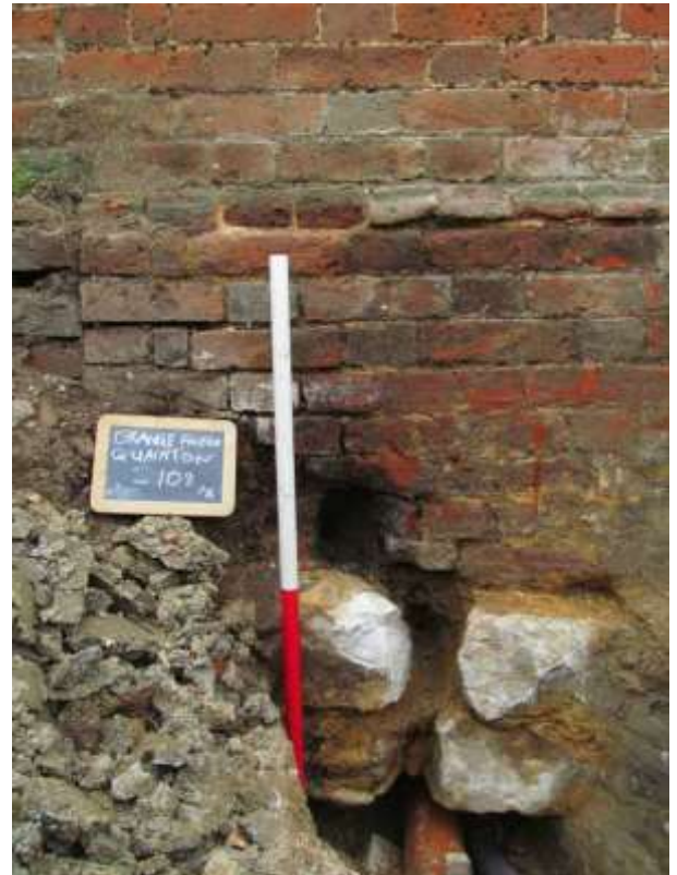
Plate 5. Section S.108, Building B4 foundations.
