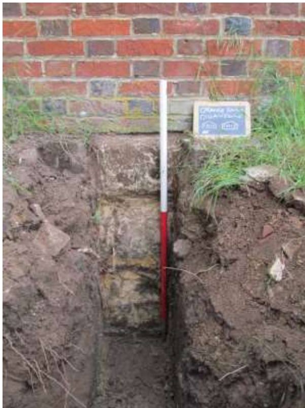
Plate 4. Section S.103, Dovecote Foundations.
