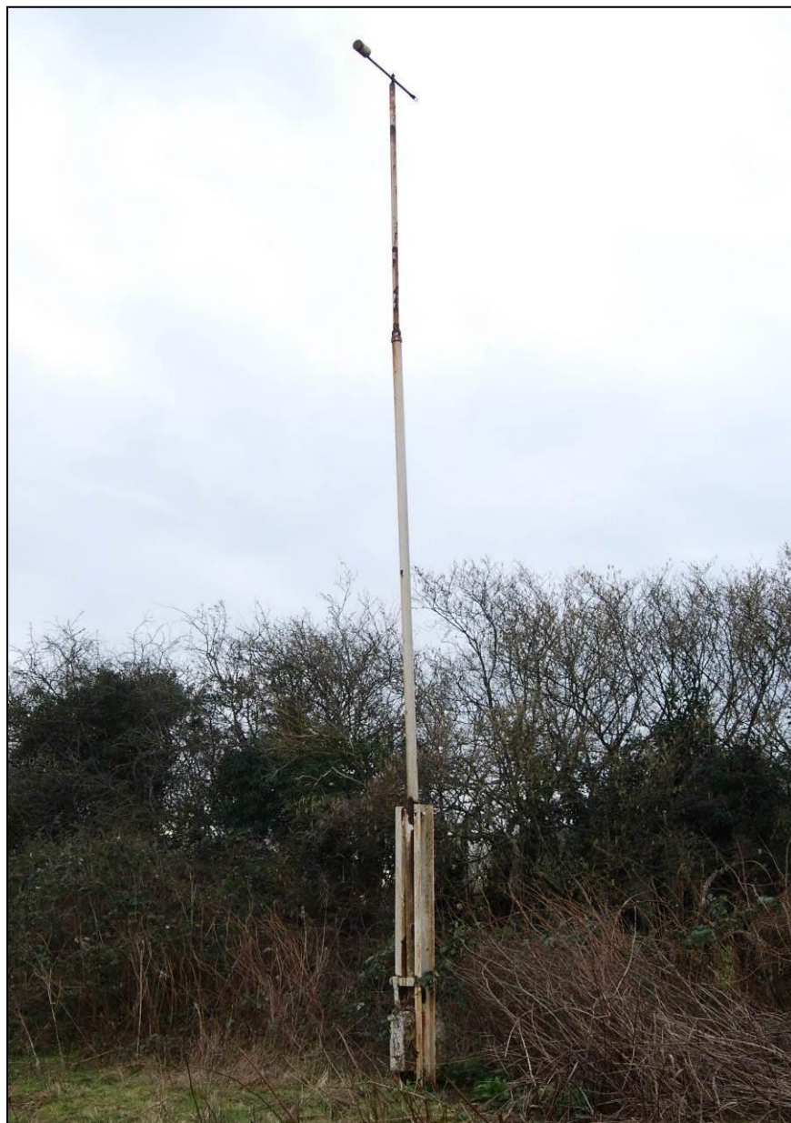
Plate 10: Windsock Pole. Looking South
