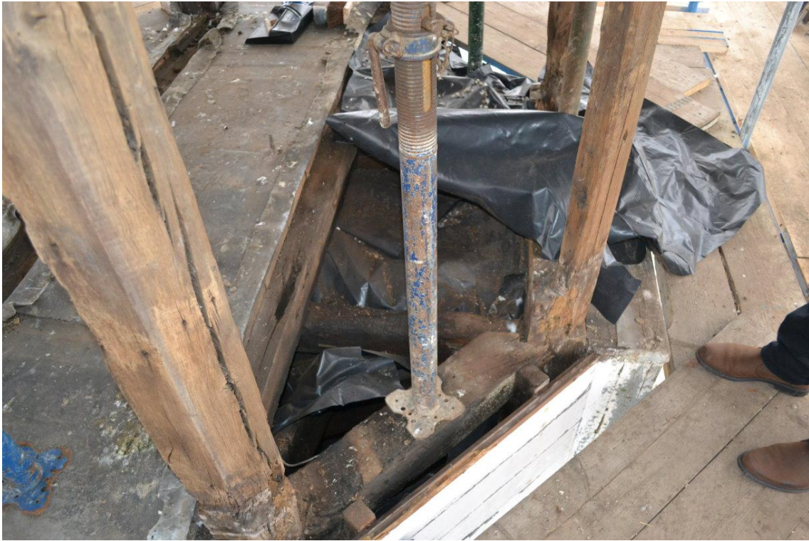
Figure 19 Base of Posts Showing Truncation (Looking East – South East).
