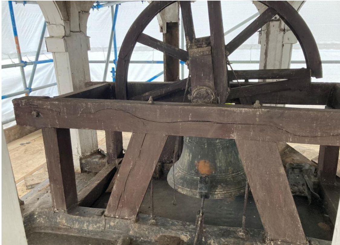
Figure 15 Bell Frame (Looking North).
