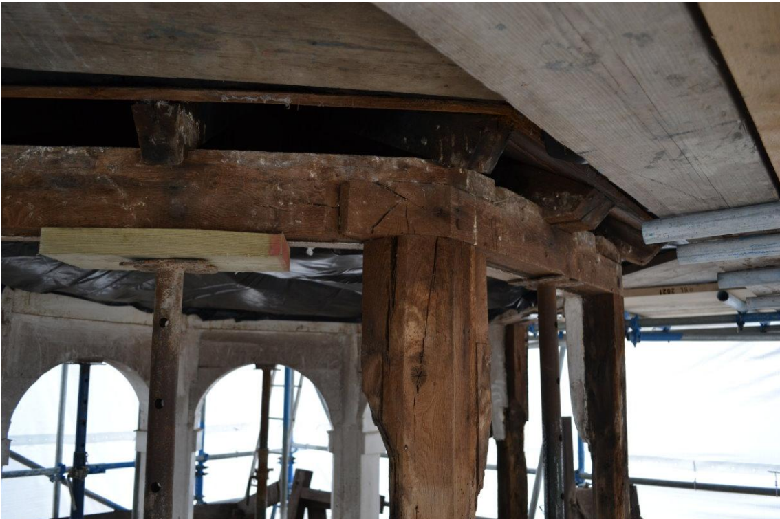
Figure 18 Clock Tower, Lapped & Pegged Wall Plate (Looking South East).
