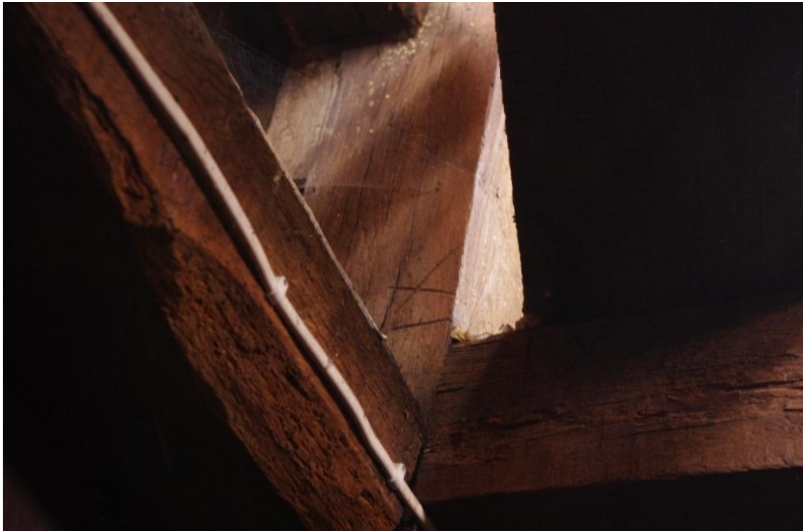
Figure 14 Inscribed Assembly Mark on Main Frame.
