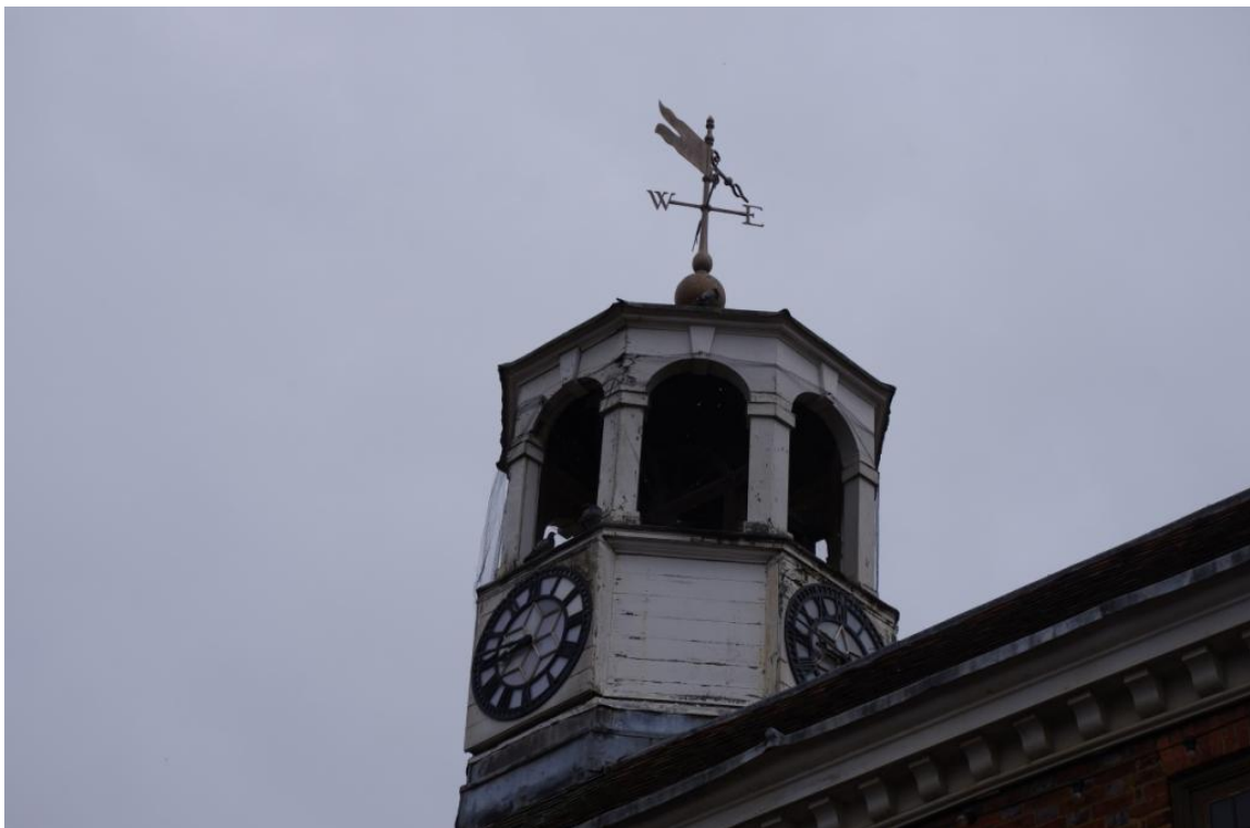
Figure 12 Clock Tower, General View (Looking North West).
