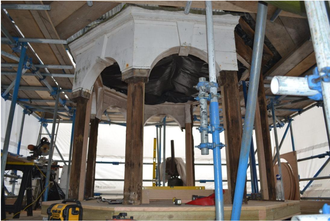
Figure 17 Clock Tower, Exposed Posts (Looking East – South East).
