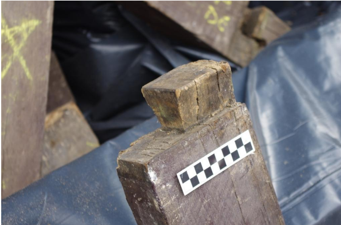
Figure 16 Dovetail Joint on Bell Frame (Post Removal).
