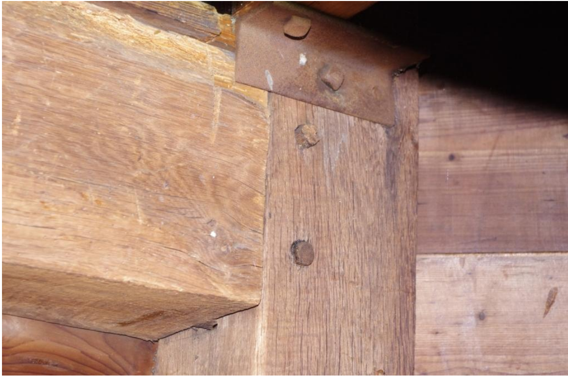
Figure 13 Pegged Frame.
