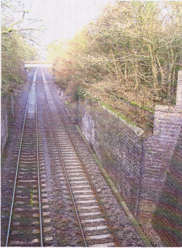
18. Base of bridge which formerly carried Wotton Tramway across the GWR line can be seen on right.
