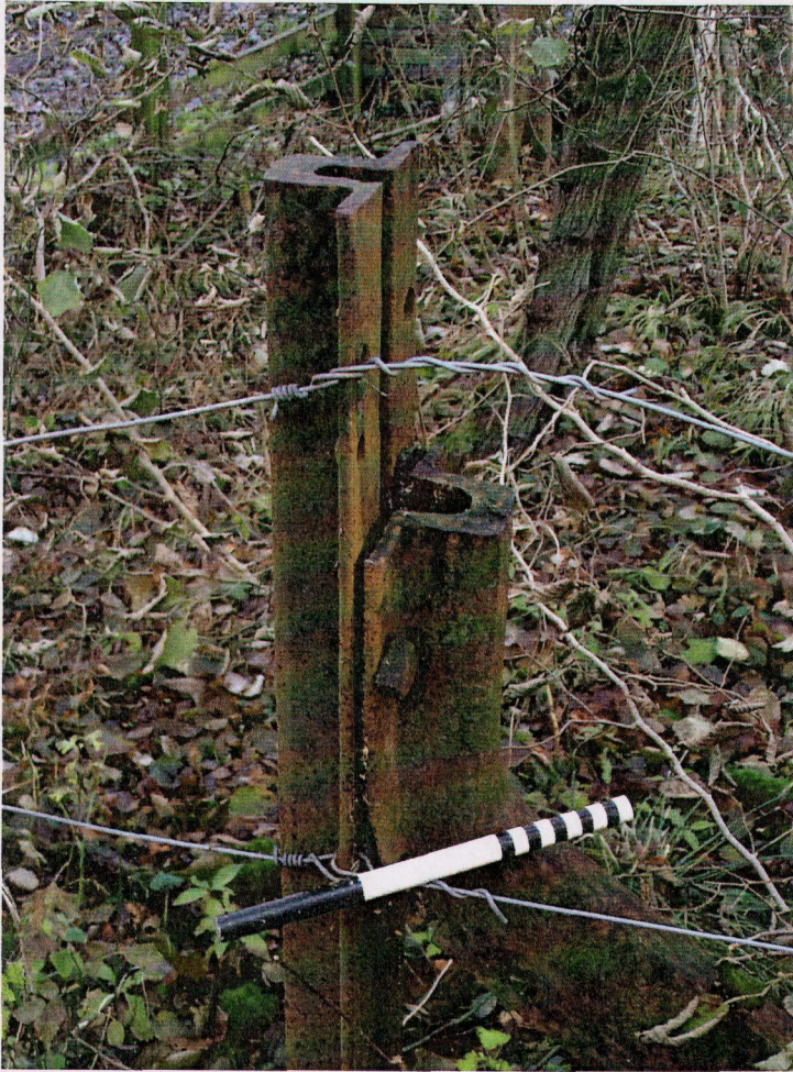
23. Bridge head rail from Wotton Tramway used as fence posts
