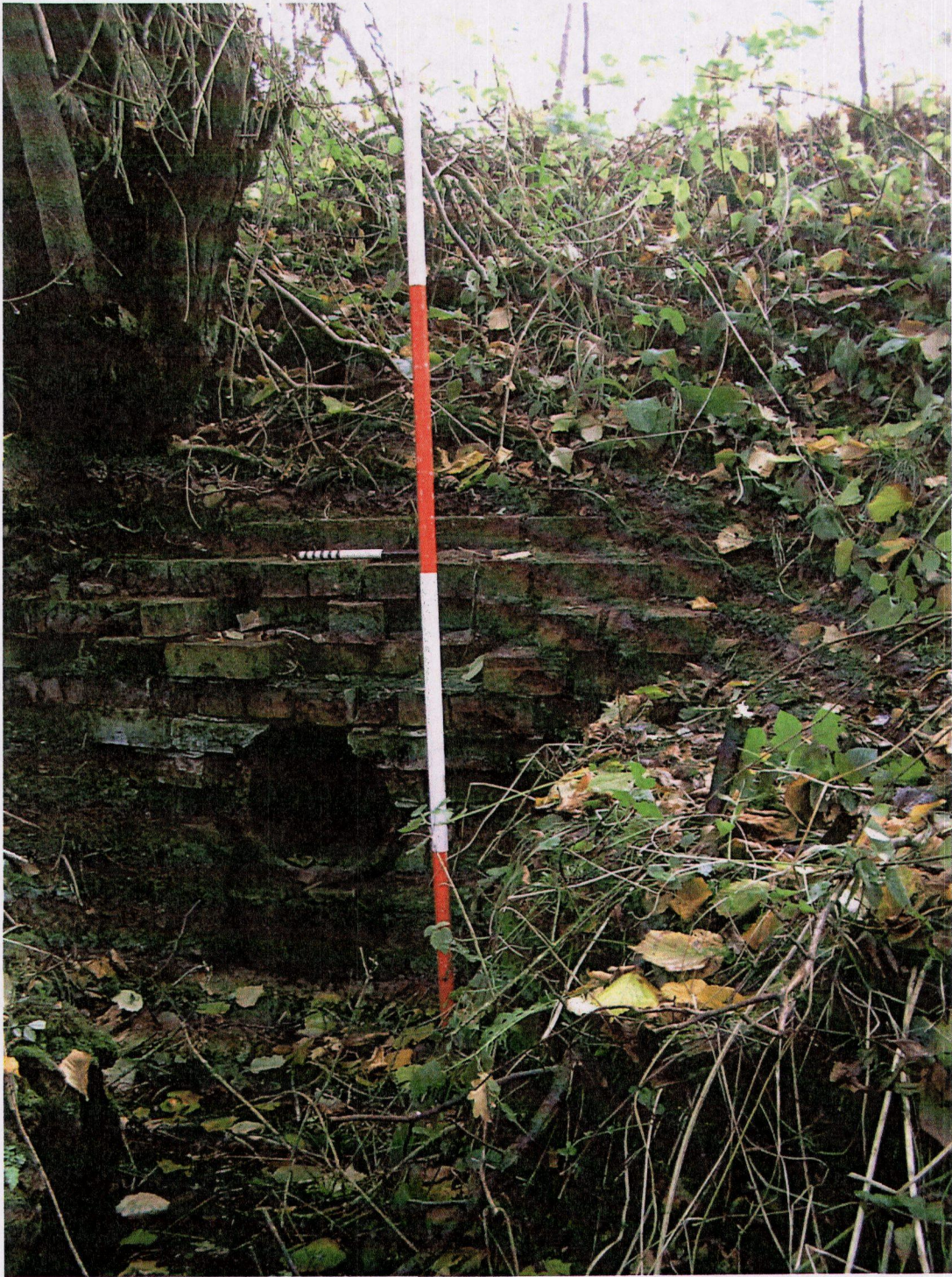
20. Culvert carrying stream beneath trackbed.
