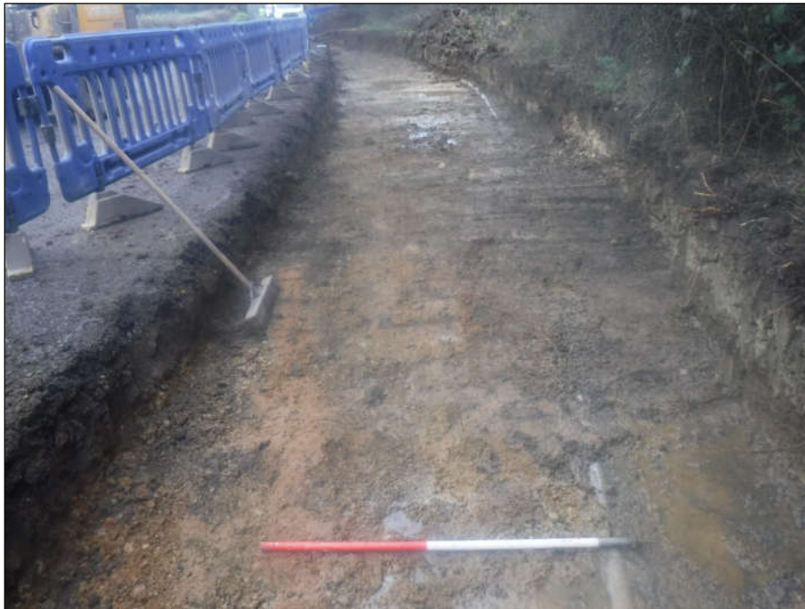
Plate 1: Post-excitation view of passing place area, looking north-east
