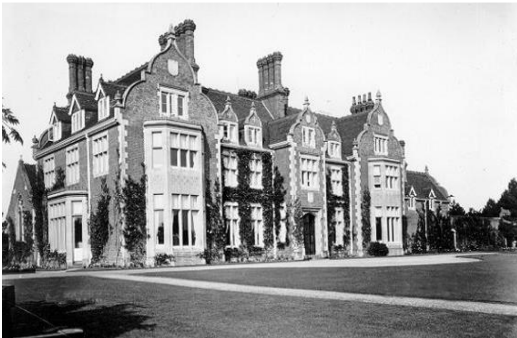
Garden front (circa 1913) chapel to the rear to left and gateway to stable yard to right.
