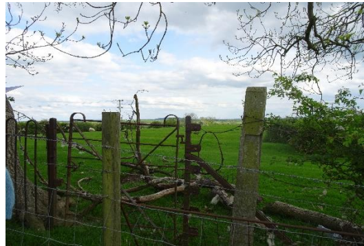
Remains of C19 iron park railing and gate on Spring Hill
