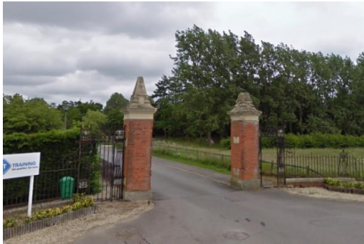
Gate piers at main entrance
