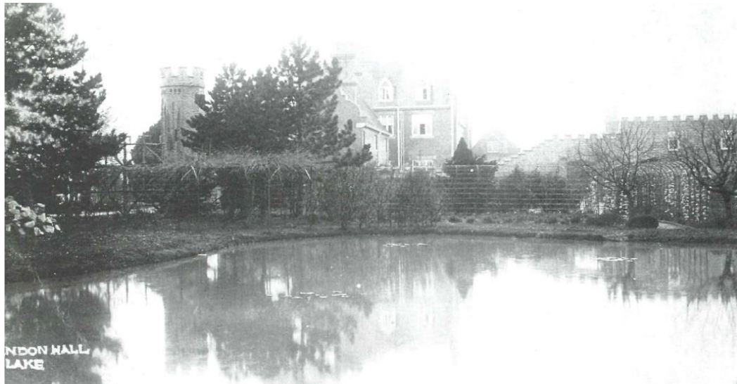
View of east side of house, across the lake, showing tower at entrance to the service yard (demolished during WWII) and tunnel arbour to the right c.1910
