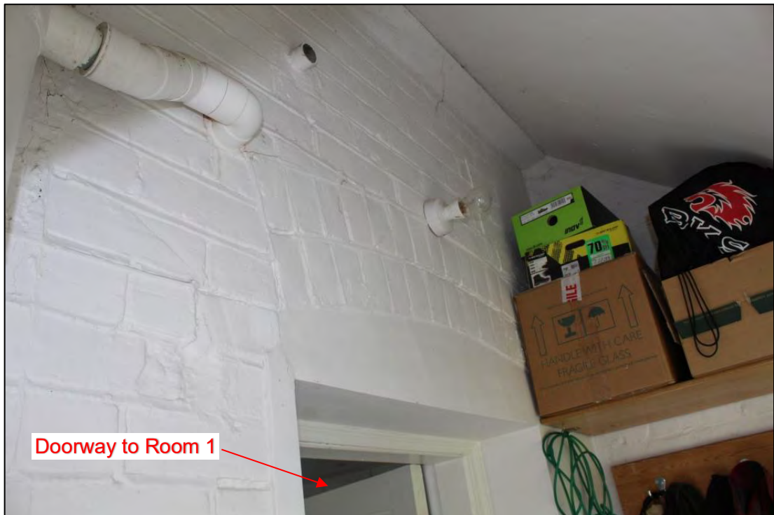
Photo 15: Detail of brickwork and segmental arch in Room 2
