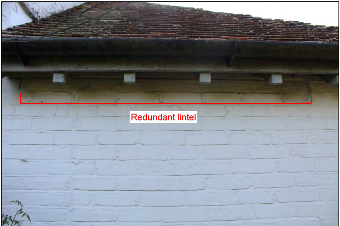
Photo 11: Detail of redundant lintel within northern elevation
