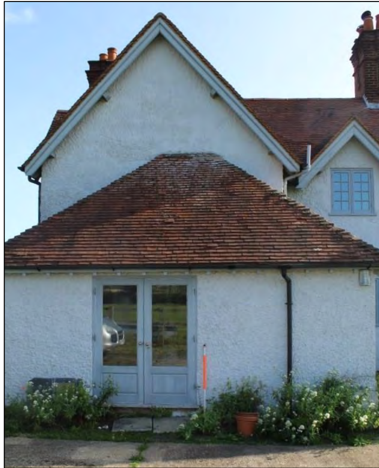
Photo 6: Northern extent of western elevation
