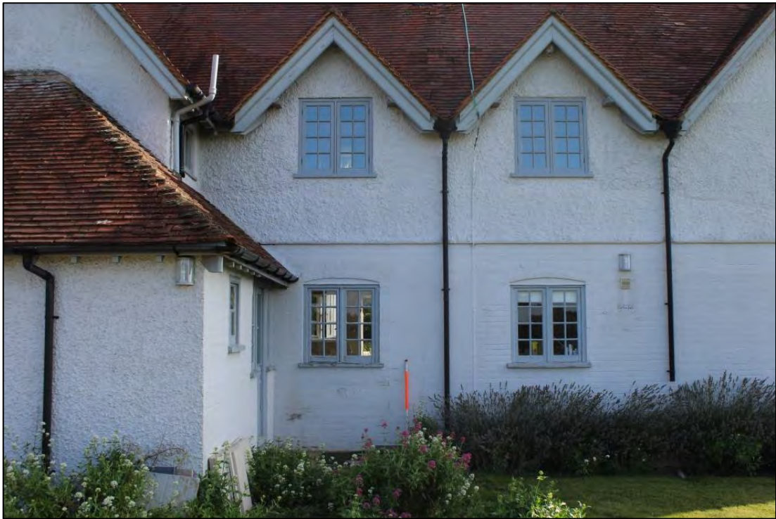
Photo 5: Central bays of the western elevation
