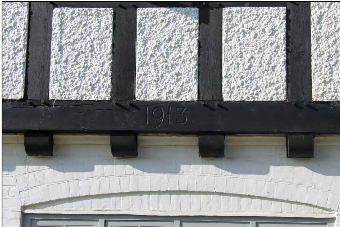
Photo 2: Carved date on northernmost gable end of eastern elevation
