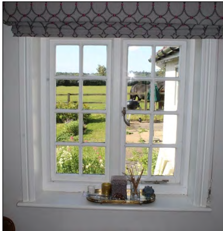
Photo 19: Detail of window within western wall of Room 4
