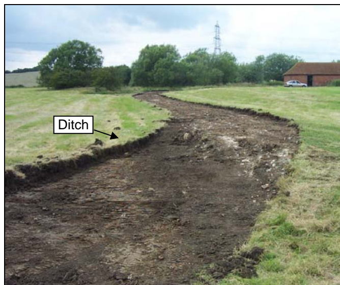
Plate 14: The existing access, showing the line of the new route.
