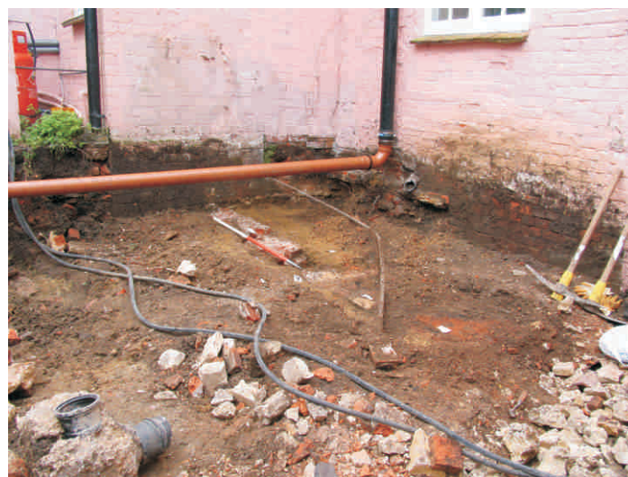
SOUTH FACING SHOT OF THE AREA OF PROPOSED DEVELOPMENT SHOWING THE INITIAL REDUCTION OF GROUND LEVEL IN THE AREA OF PROPOSED DEVELOPMENT.
