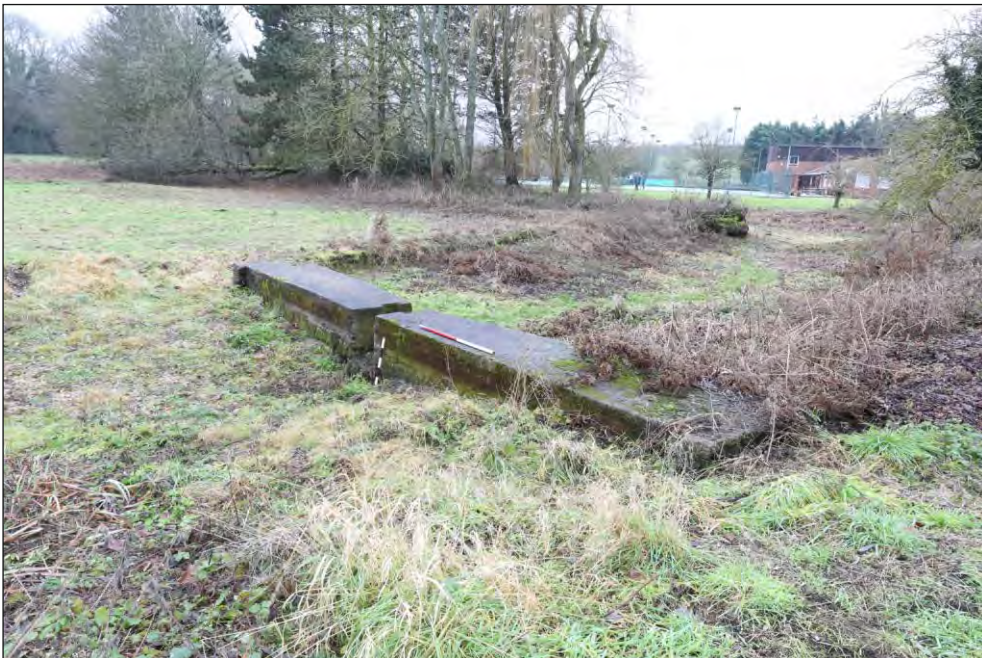
Plate 8: Weir 2, viewed from the north-east
