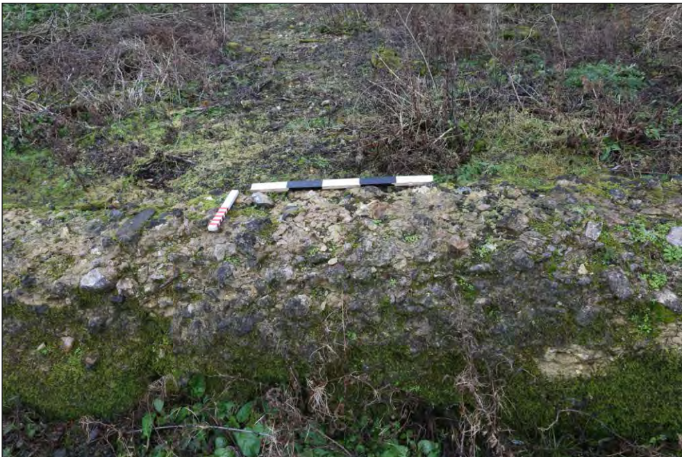
Plate 6: Detail of the fabric of Weir 1, viewed from the south-west
