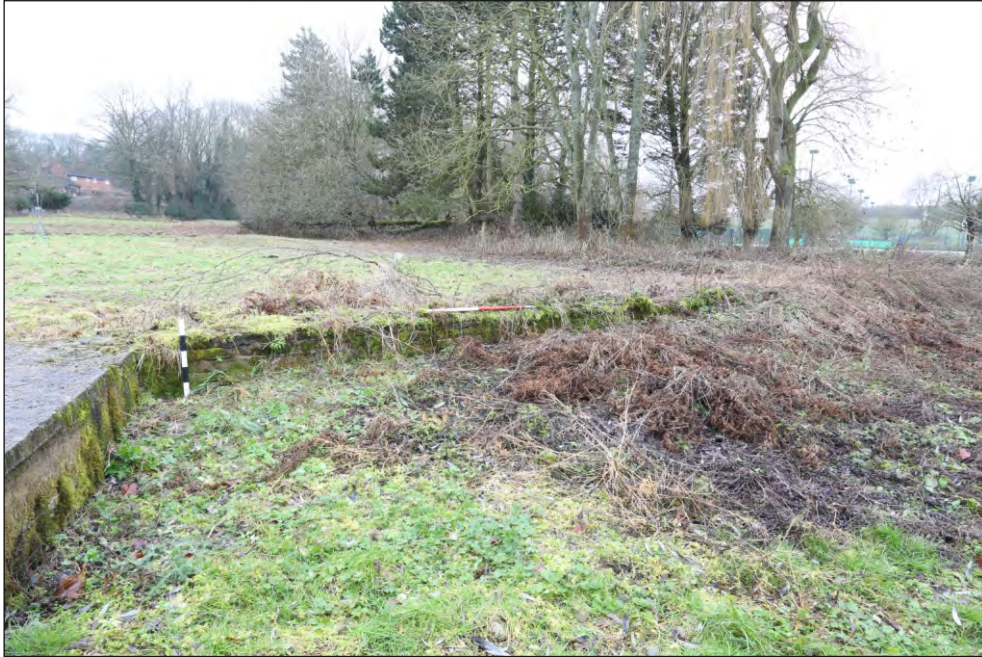
Plate 9: The wing wall of Weir 2 viewed from the north-east
