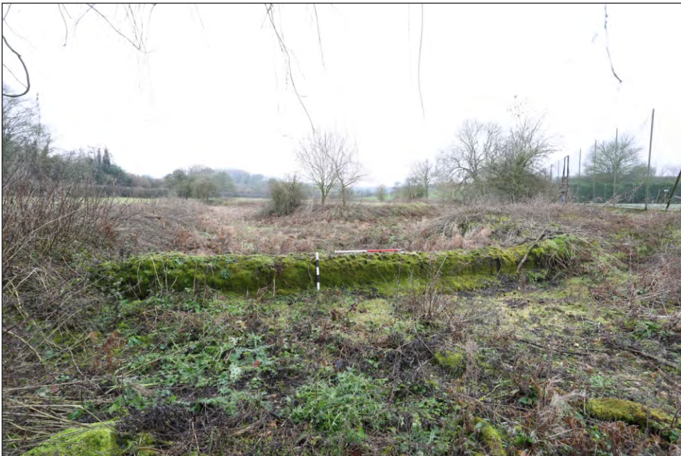
Plate 4: Weir 1, viewed from the north-east
