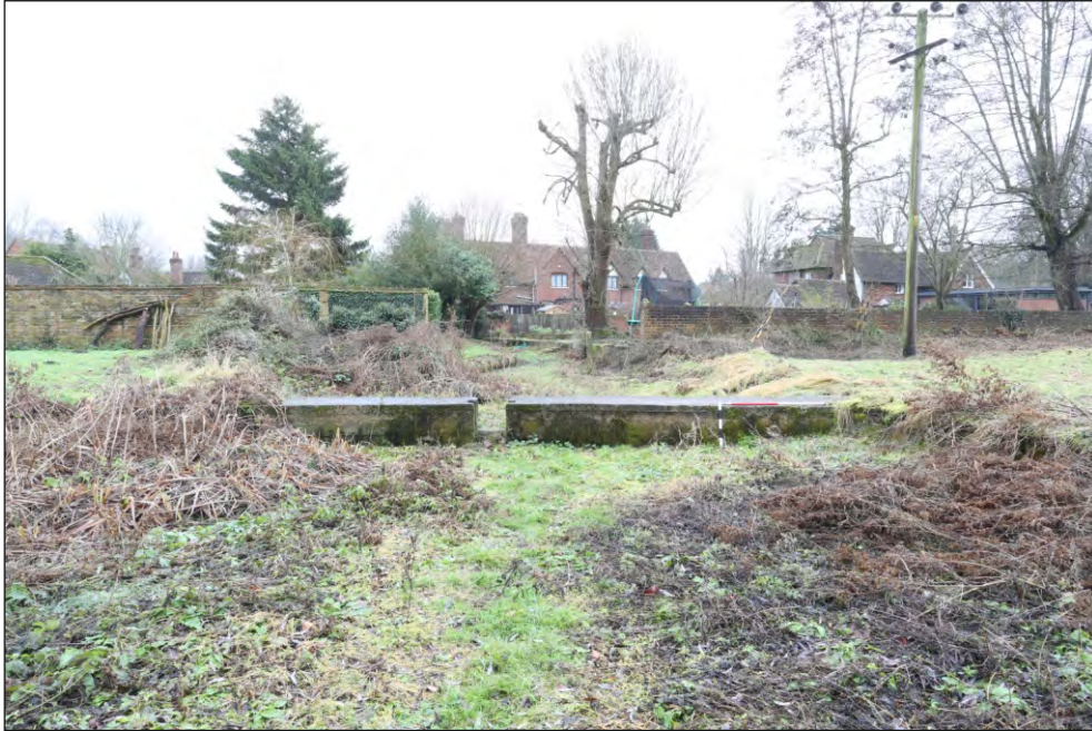
Plate 7: Weir 2 viewed from the north-west
