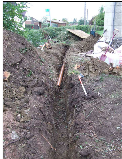
Plate 11: General view of service trench 1, looking NW ( scale 2x1m )
