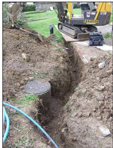
Plate 15: General view of service trench 4, looking NE (scale 1m)
