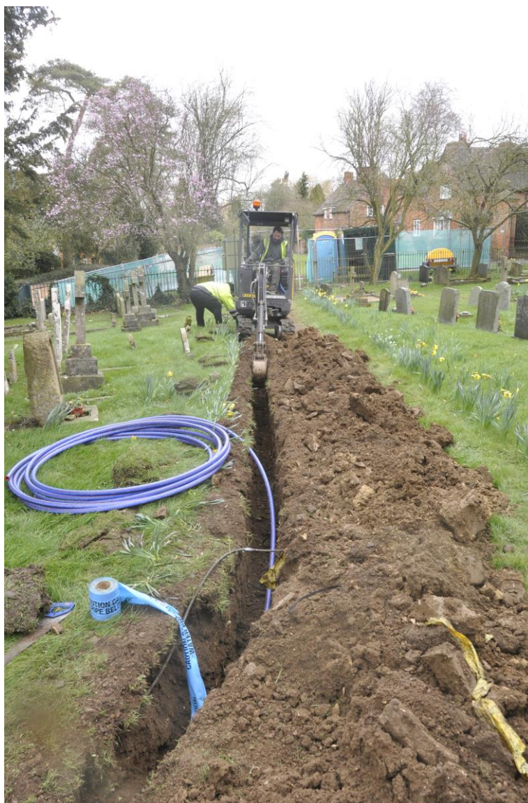
Plate 1. Service trench under excavation. View to north.
