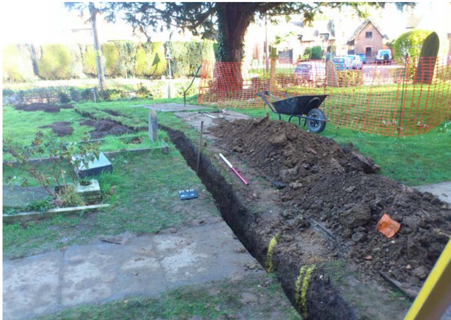
Plate 1. Pipe trench, looking north from church towards graveyard.
