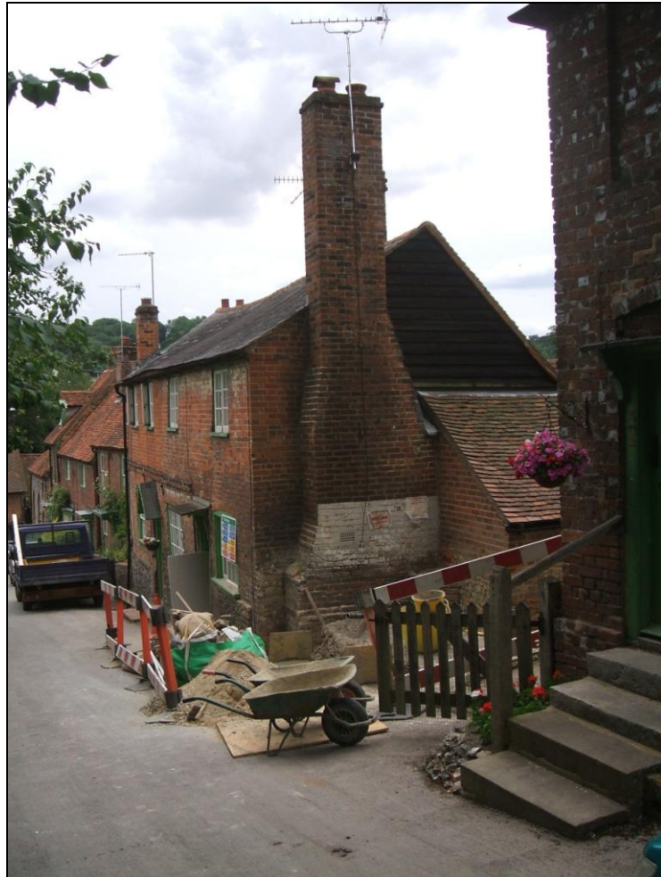
General view of the excavation area, looking south-west
