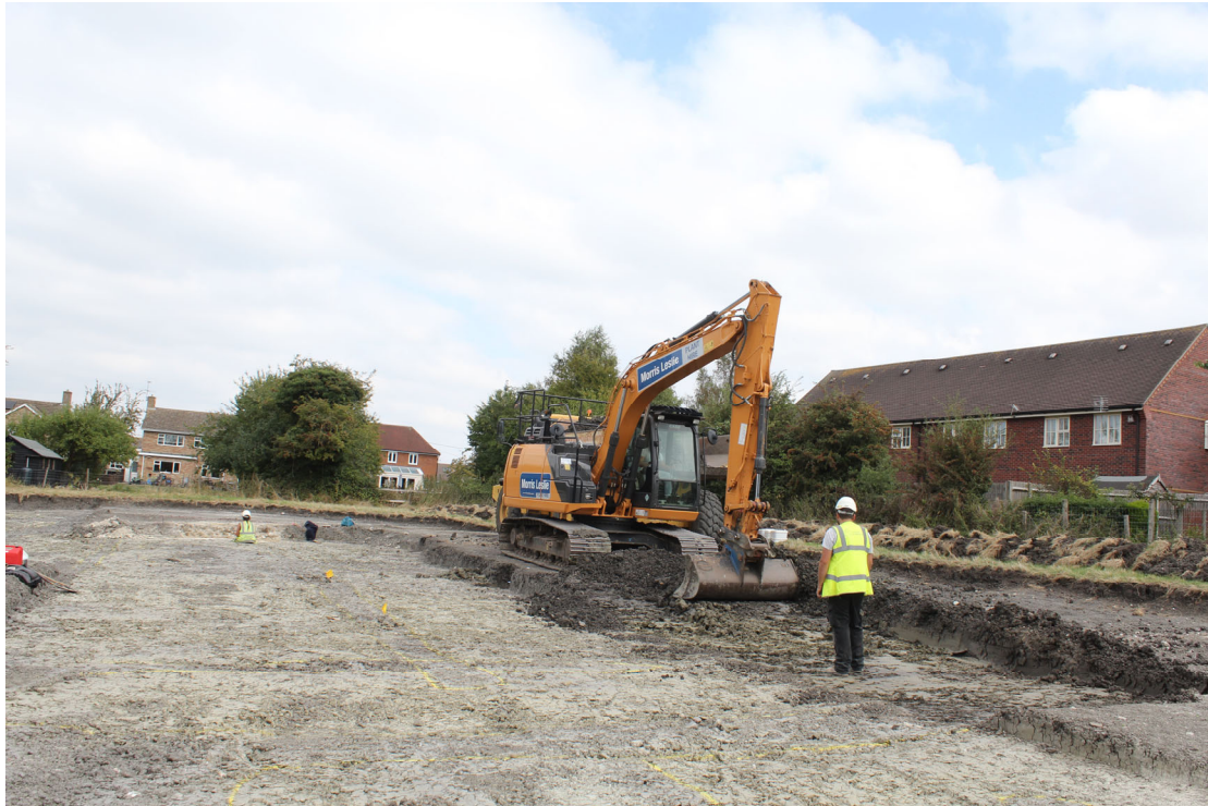
5 - Garden Soil 2003 under excavation
