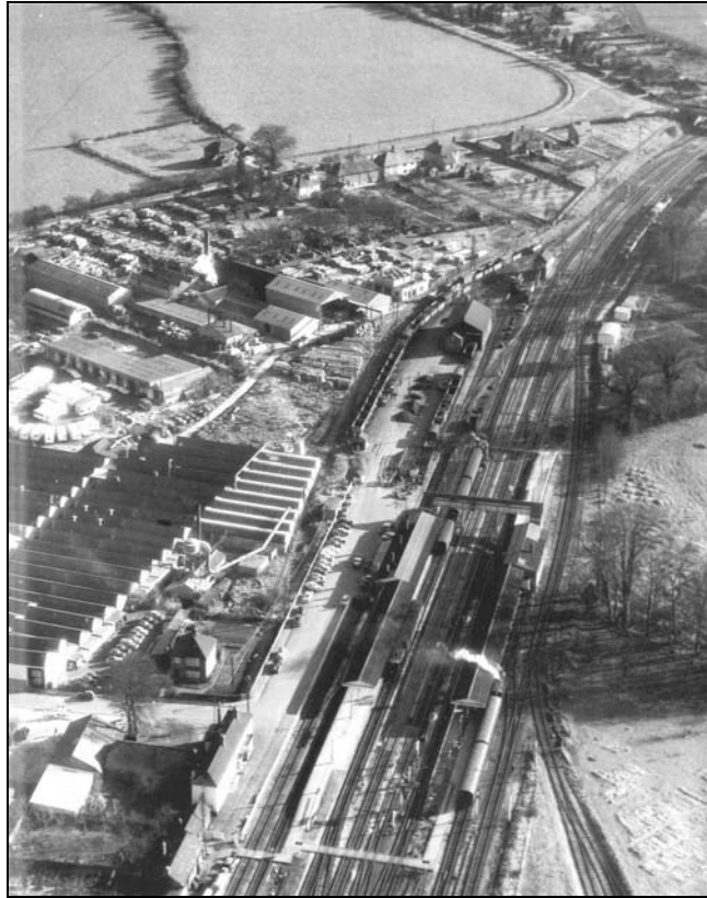
Plate 10: View of the furniture factory 13 th March 1959
