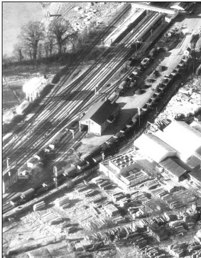
Plate 11: View of the timber yard 13 th March 1959
