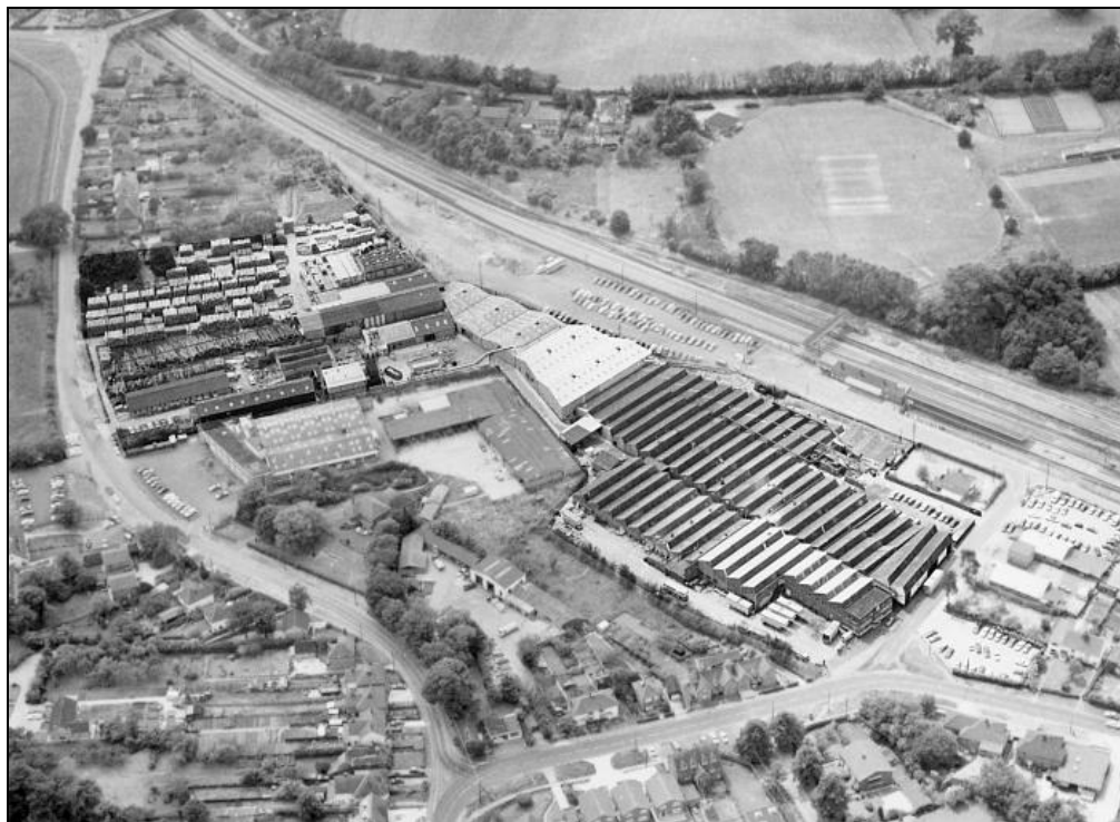
Plate 13: Aerial view of the assessment site in 1973
